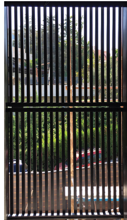
Vertical Aluminum Profiles On Aluminum Frame
