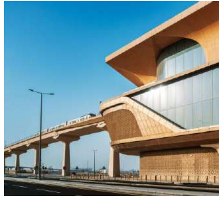
Gold Line Metro, Doha
